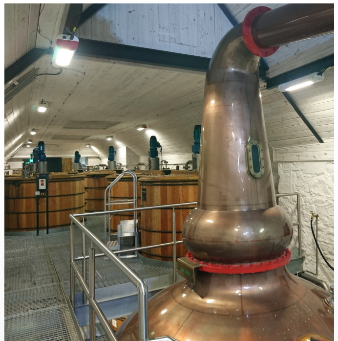
Torabhaig is a traditional farm steading and croft, now converted to a modern distillery. A mixture of SPARTAN Zone 1 and Zone 2 luminaires were installed, all painted in white to blend in with the wood panelling which was already in place.
